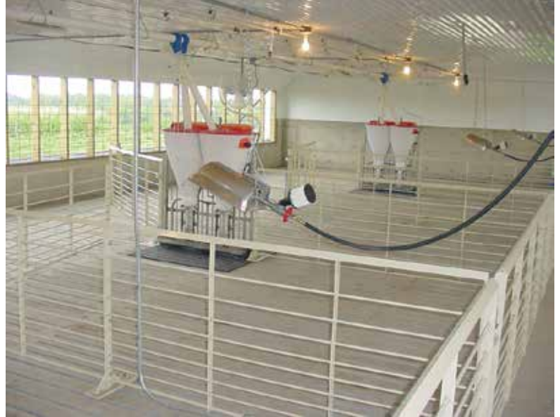
Typical installation of Gasolec M5 in a Hog Barn
